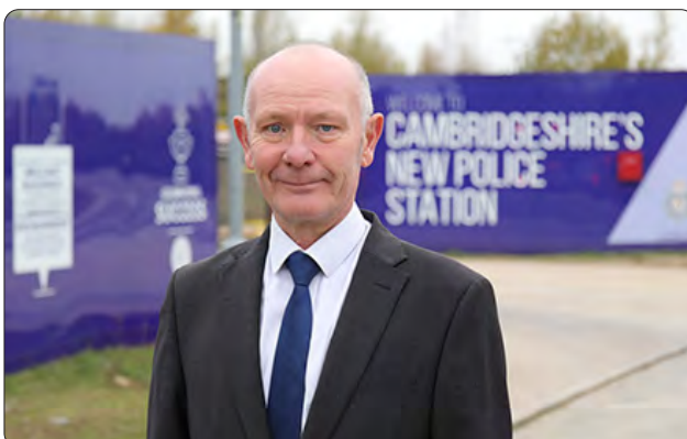
Commissioner Darryl Preston at the site of the new Cambridge police station in Milton; it is due to become operational during 2026.
